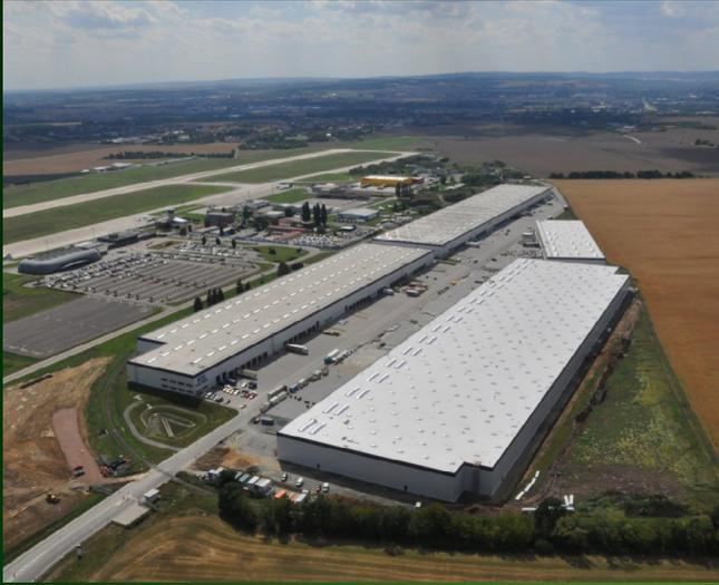
Brno Industrial Park consists of a developed area of 109,457 m<sup>2</sup> in total. It is a unique multi-purpose zone with buildings designed to have the lowest possible impact on the environment. Part of the area was built on a brownfield and up to 90% of the materials obtained from demolition of the original buildings were used in the construction. The multimodal complex neighbouring with Brno Airport was constructed by Brno Airport a.s., a company of Accolade Group.
